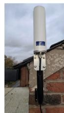
Once the bolts are fitted and the antenna is secured, feed the cable through the pre-drilled hole in the wall and affix the antenna to the wall using a 10mm Spanner.
