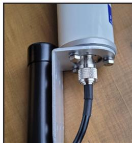
Then use the two U-bolts to fix the antenna mounting bracket to the pole using the outer holes on the antenna mounting bracket and a 10mm spanner. Ensure that the washers are used and bolts are not over-tightened.
