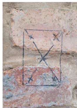
Normal masonry wall plugs and screws or another alternative can be used ( not supplied ) depending on application. Once all holes are drilled, use a hammer to knock the expansion bolts into the holes ready for applying the bracket.
